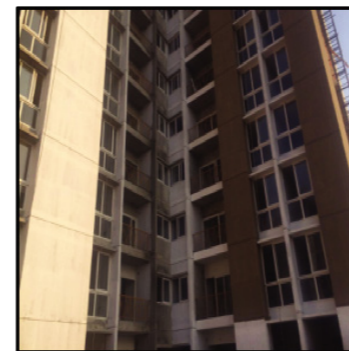
Tower C - C1 & C2 section upvc work is under progress.
