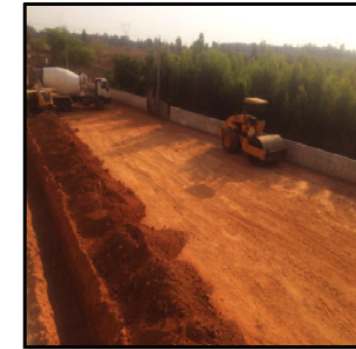
Tower C - West side filling work is in progress.
