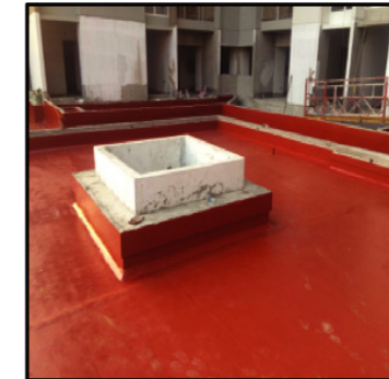
Tower - C Podium waterproofing work is in progress.
