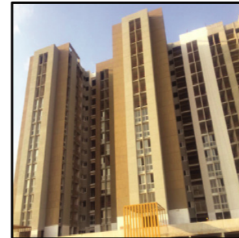
Tower C - C1 & C2 section external painting work is in progress.
