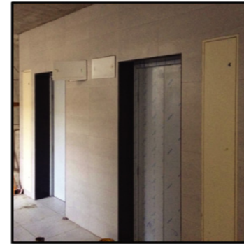
Tower C - C1 section lift cladding work mock-up
