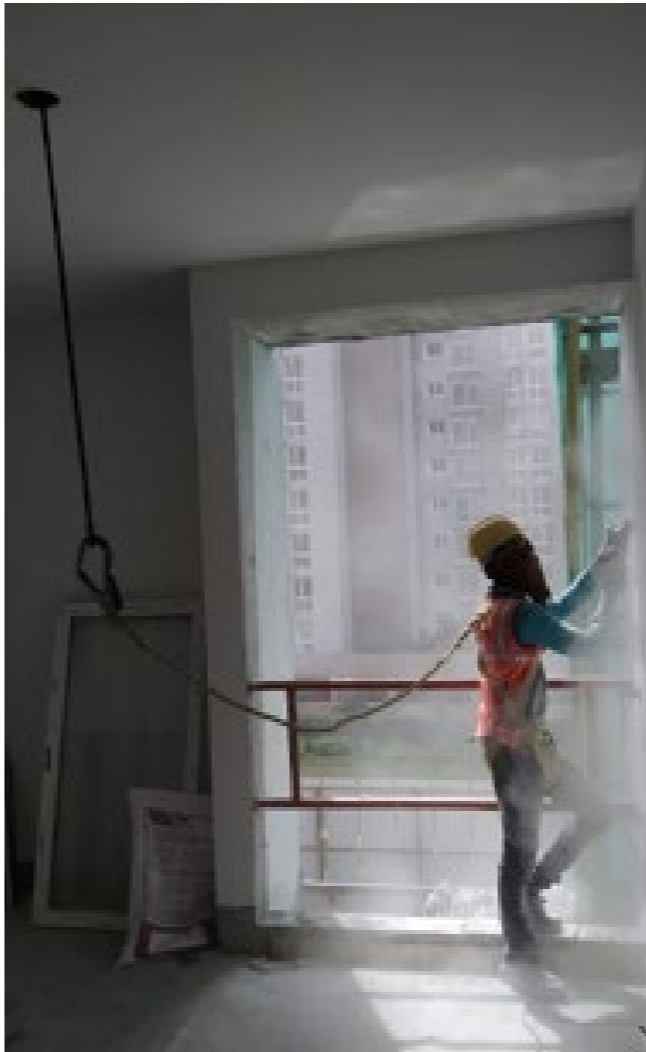
Fall arrester system implemented for grinding & painting work at building edge
