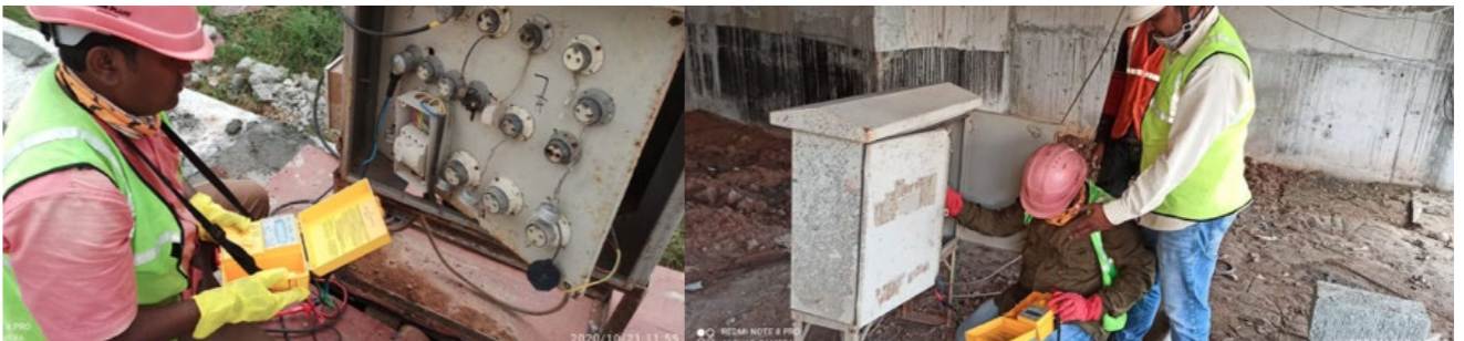
Electrical safety - RCCB/MCB Testing
