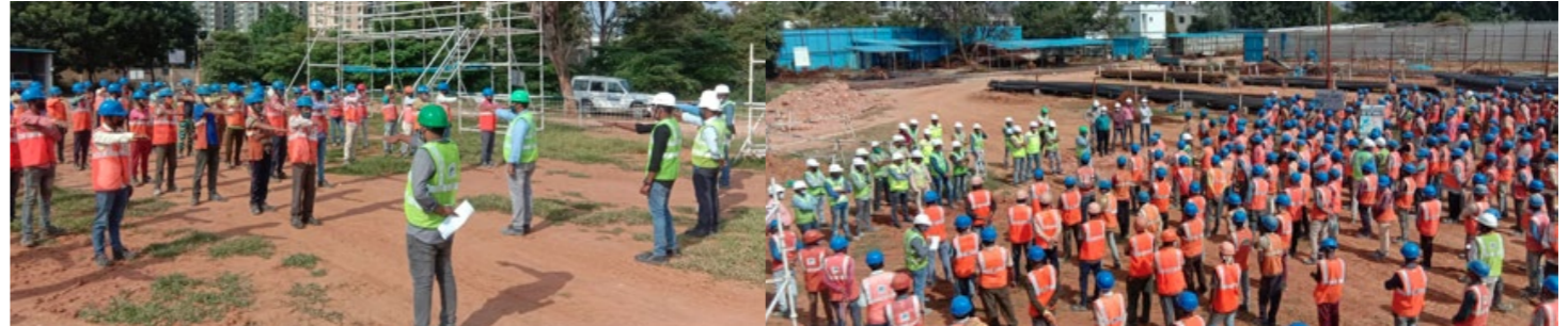
Building 2 and 3 - Everyday mass toolbox safety talk is conducted to motivate workers to follow standard protocol of safety culture.
