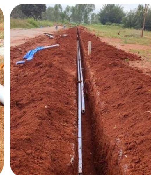
Hume Pipe Erection
