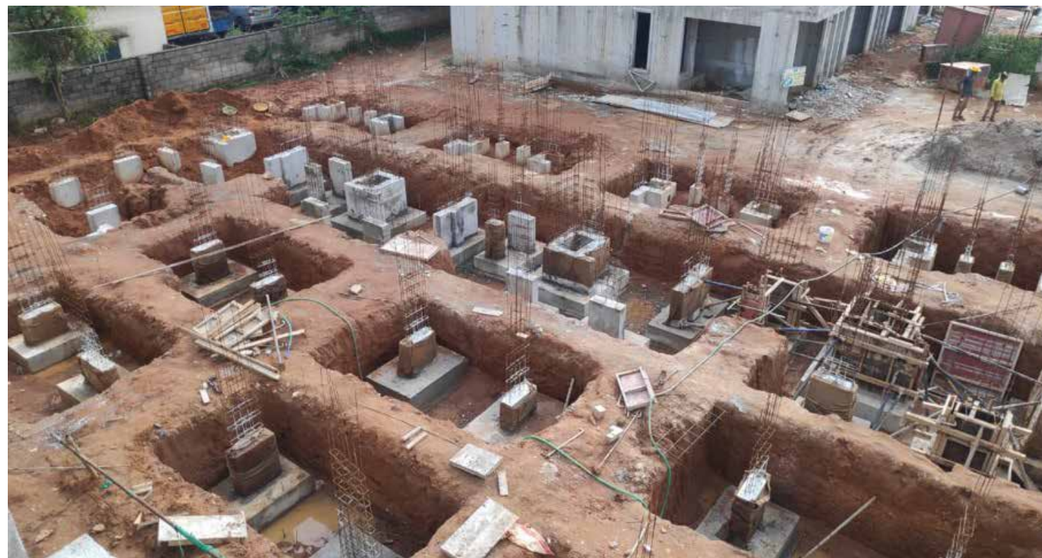
Phase 2A - The footing work in Block J8-15 is in progress.
