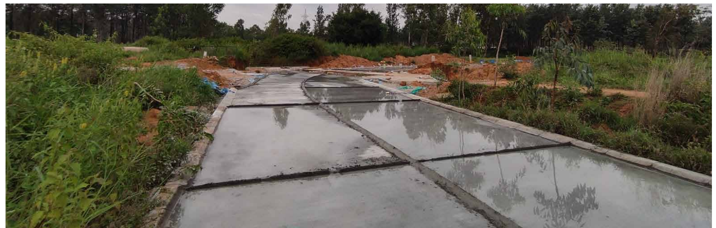
Infra Road Work - Phase 3
