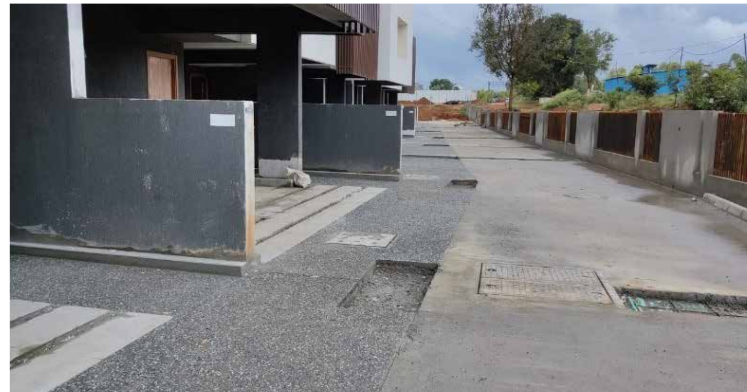
Internal Road in front of Building 6
