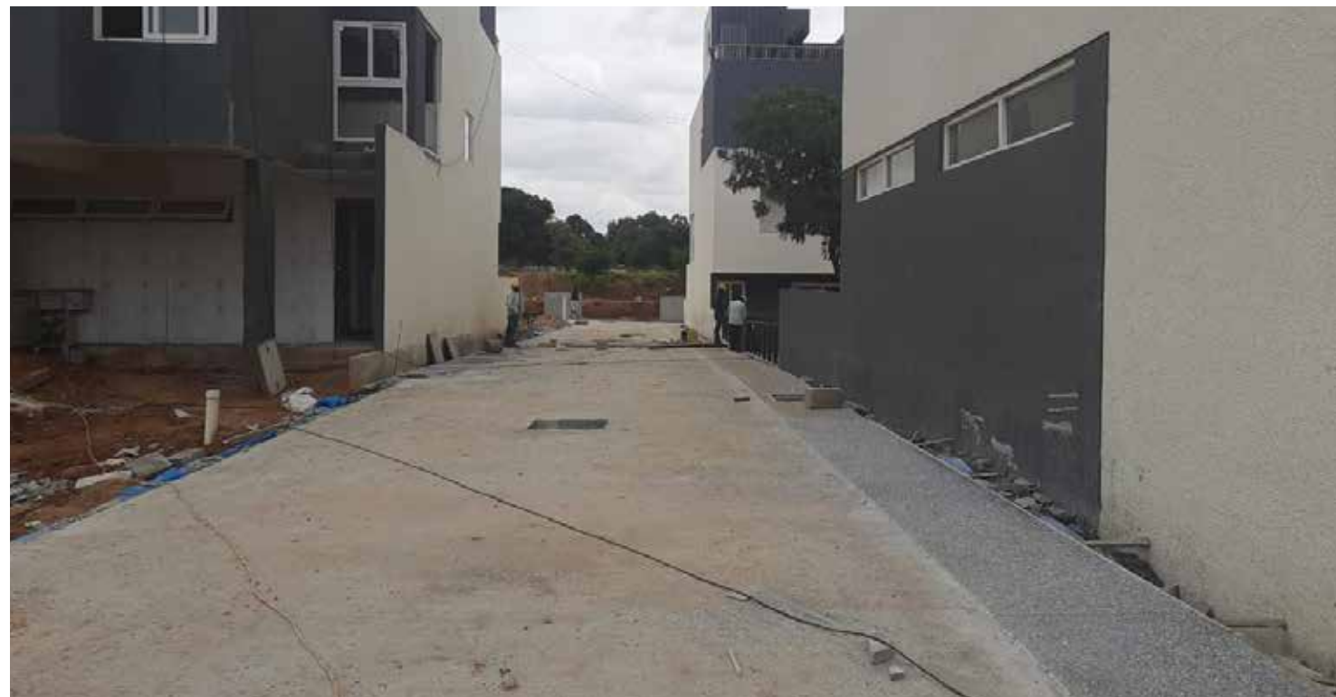
Internal Road between Building 7B & Building 3
