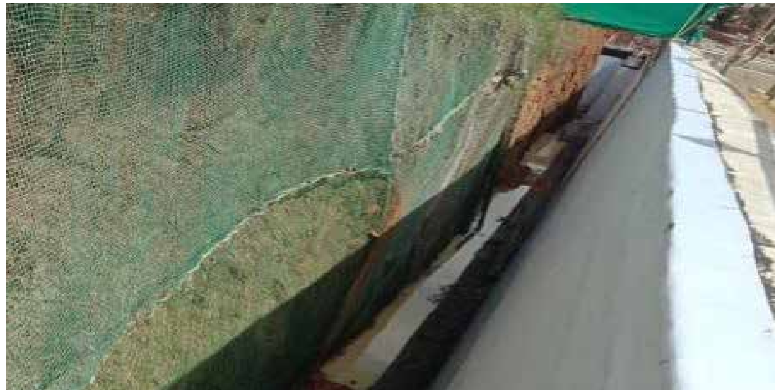
INFRA MEP WORK
