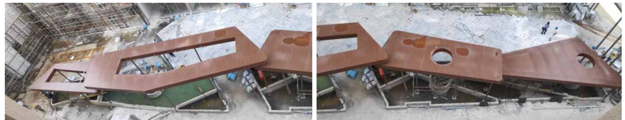
The quadrangle roof ACP work has been completed.
