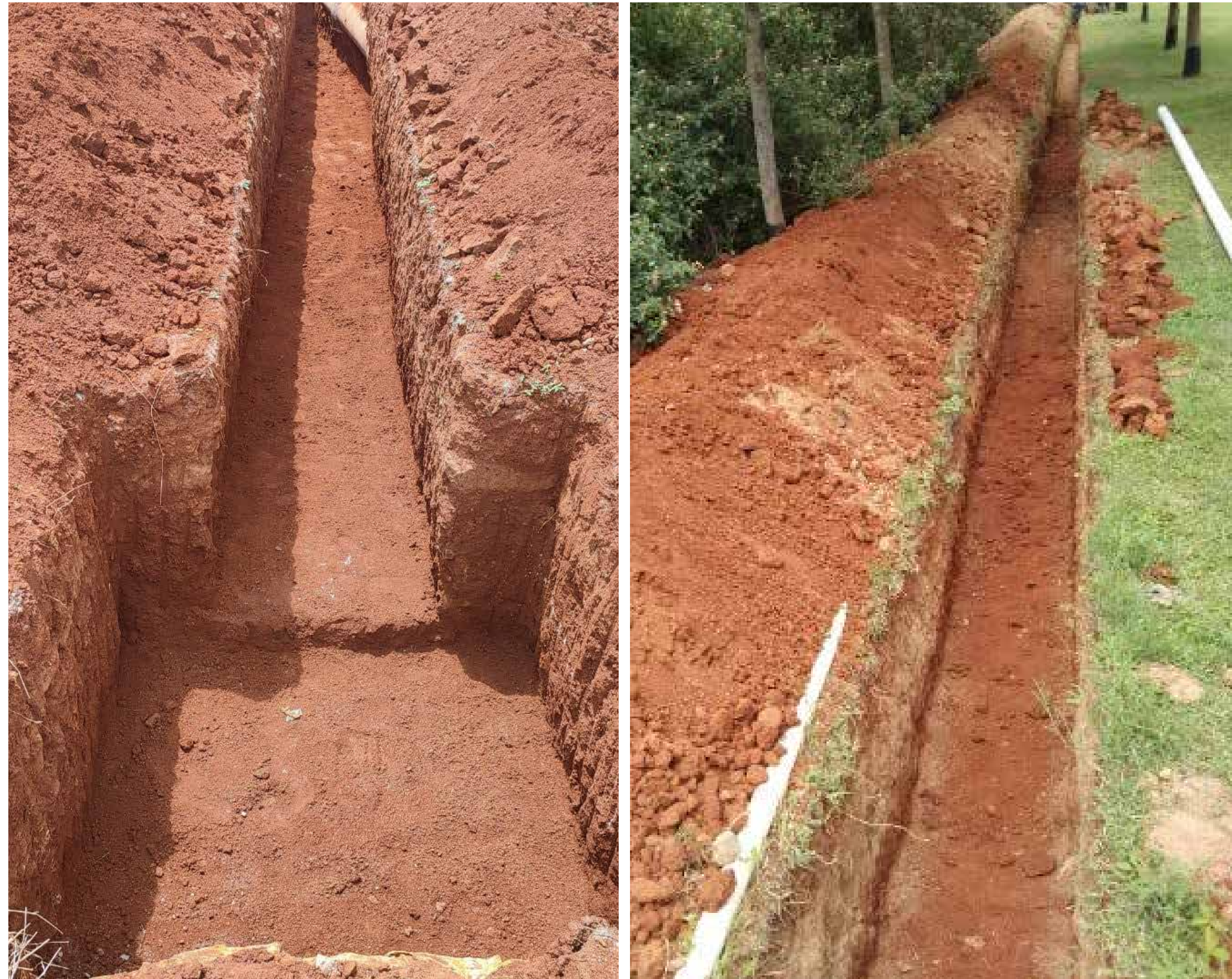
Infra MEP Work
