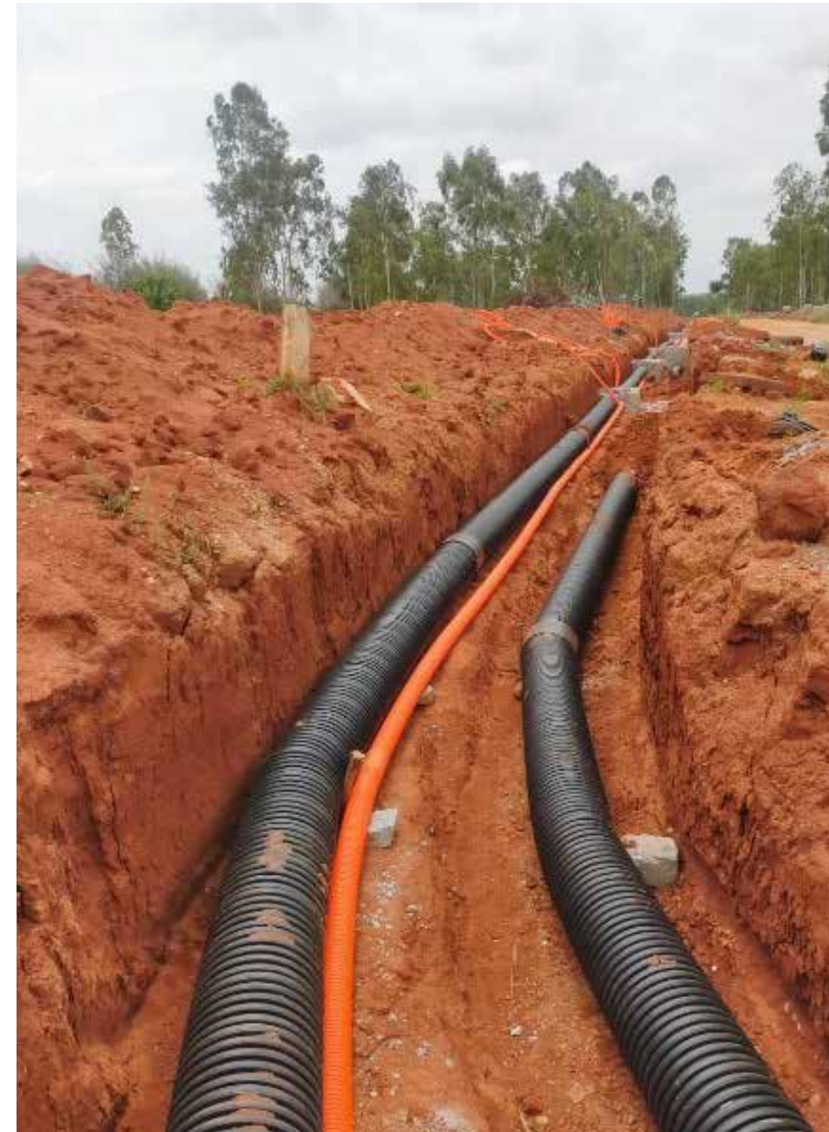
Plumbing & Electrical Infra Work
