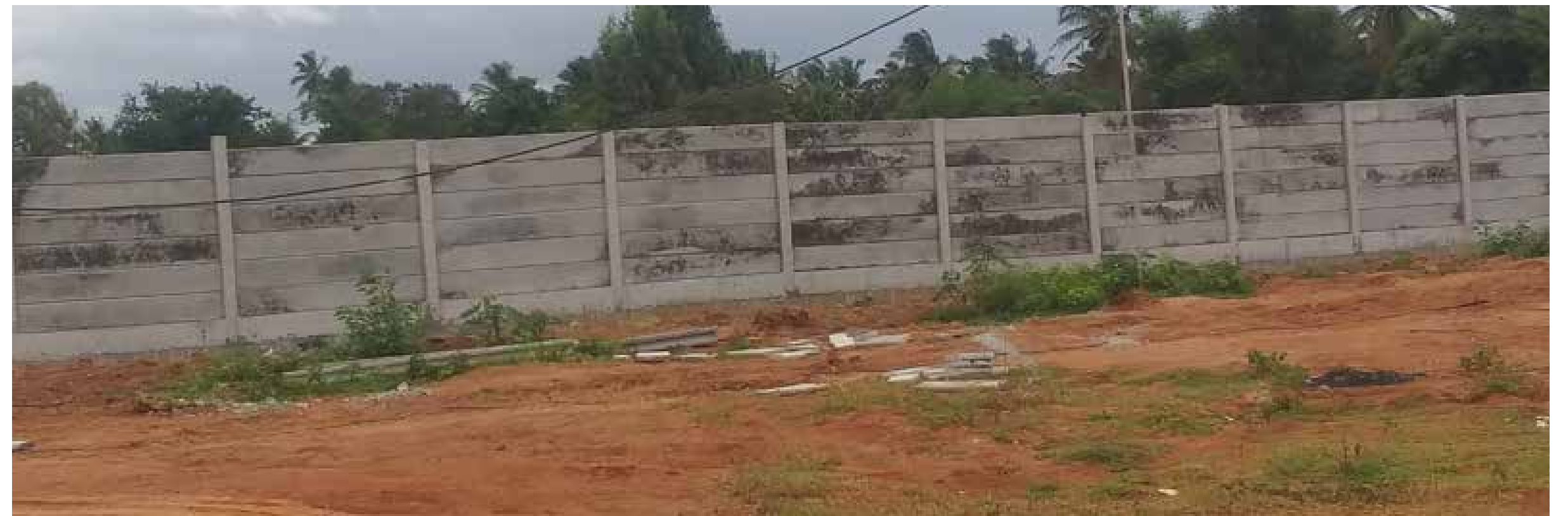
Phase 3 - Precast Compound Wall
