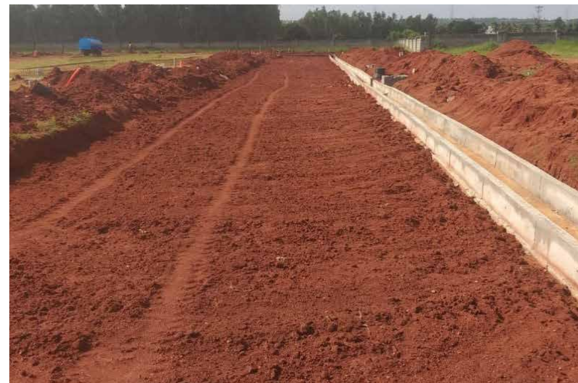
Subgrade For Roads – Phase 1
