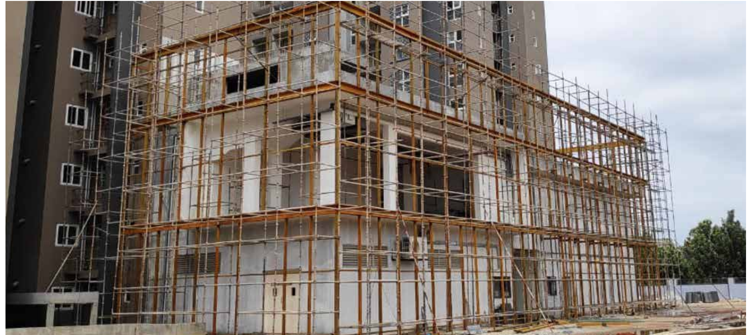
The clubhouse elevation glazing MS support work has been completed.
