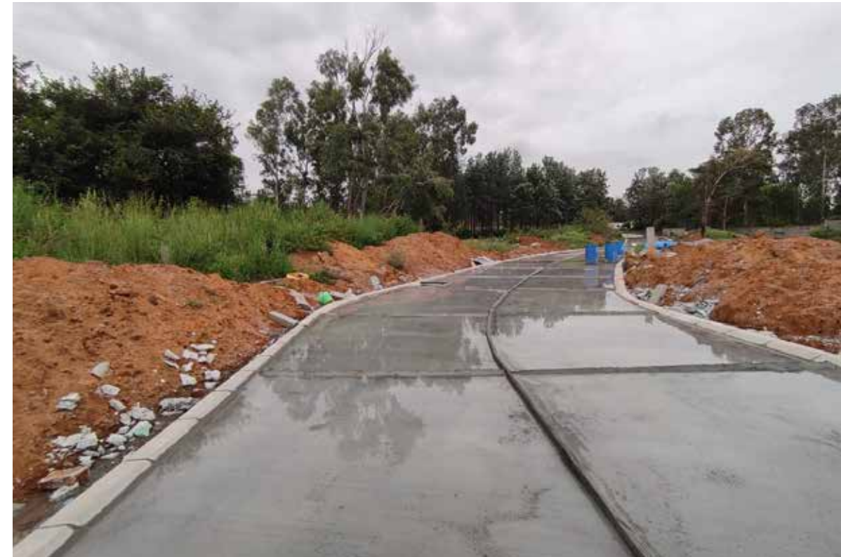
Infra Road Work - Phase 2
