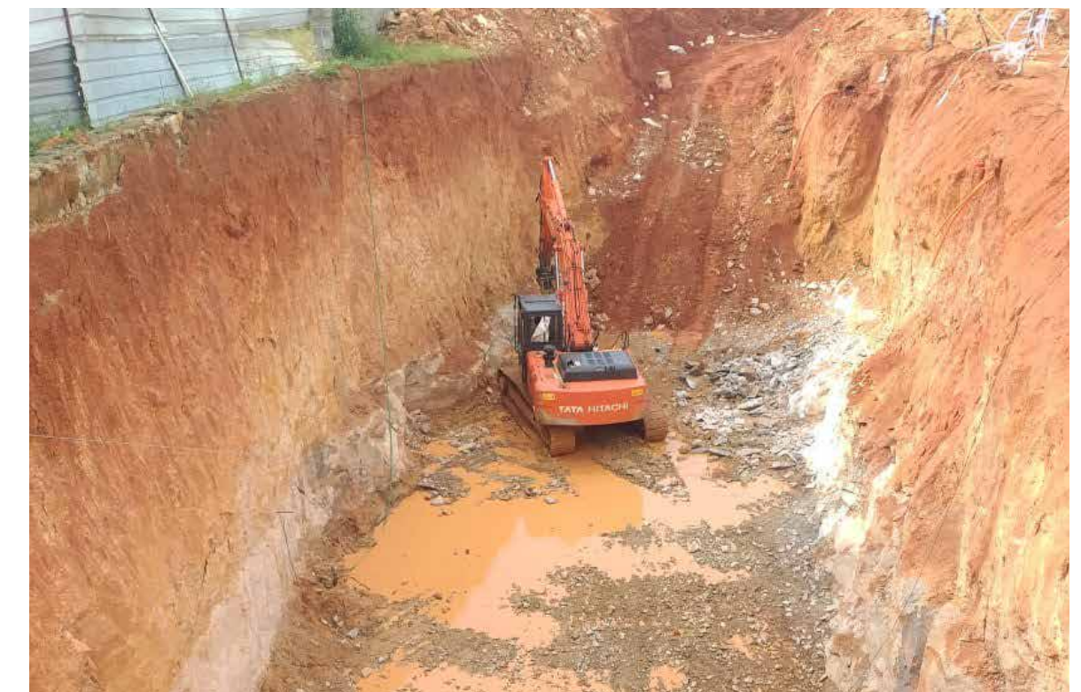
STP Excavation Completed
