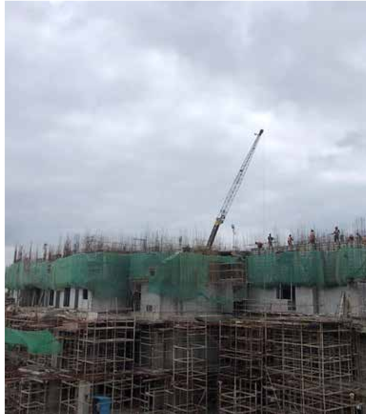
Phase 2 Building-02 - Southwest View
