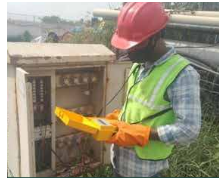
RCCB & Earth Bit Checking
