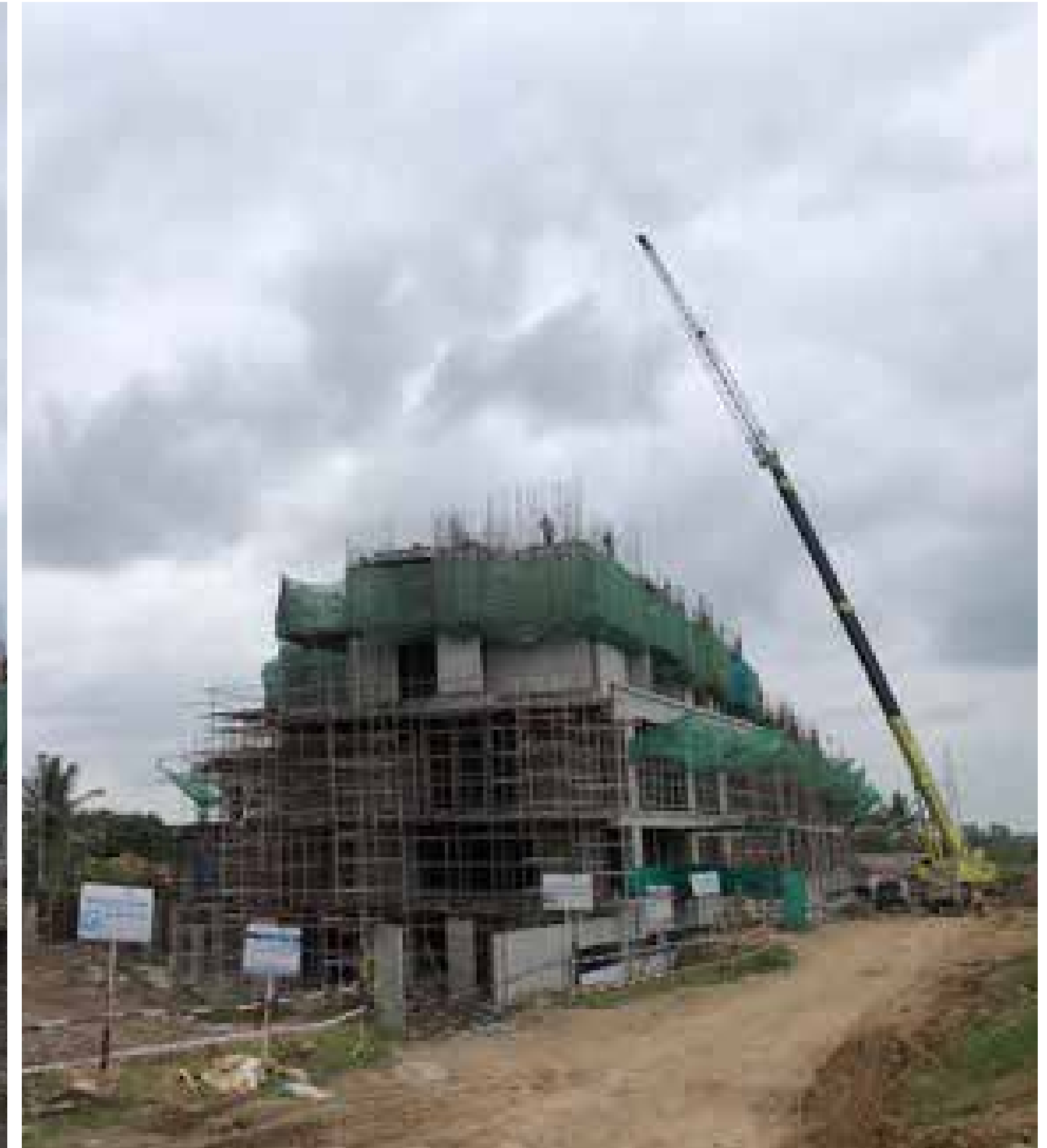
Phase 2 Building-02 - Northwest View
