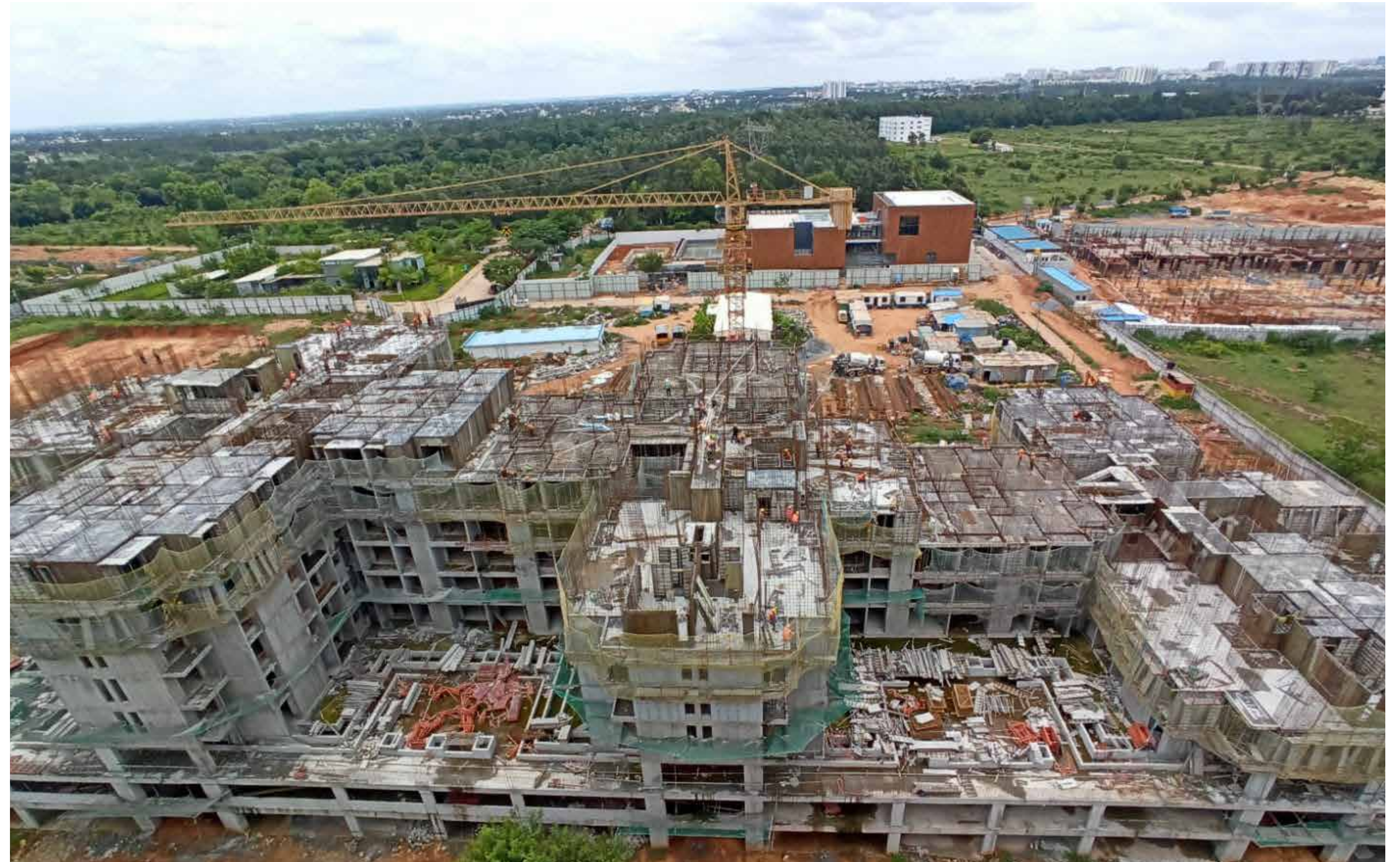
Tower B - B1, B2 & B3 Block Aerial View
