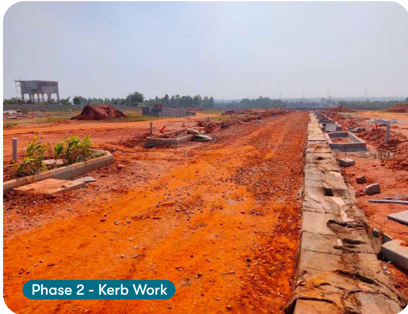
Phase 2 - Road 1st Layer Subgrade Work
