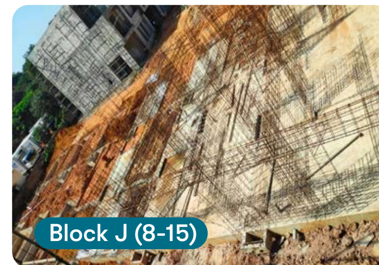
Phase 2A - Superstructure Work
