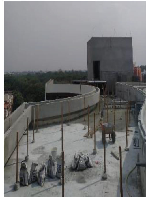
The terrace level swimming pool and amphitheatre works for Block A, B, C, & D are in progress. The lift work is in progress.
