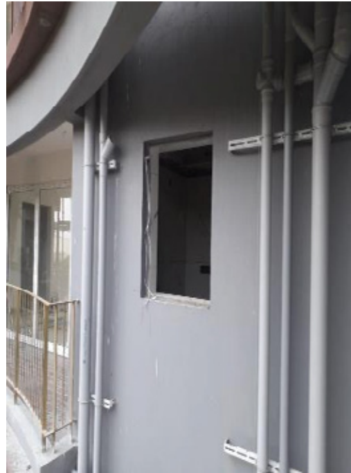
The shaft PHE work is in progress.
