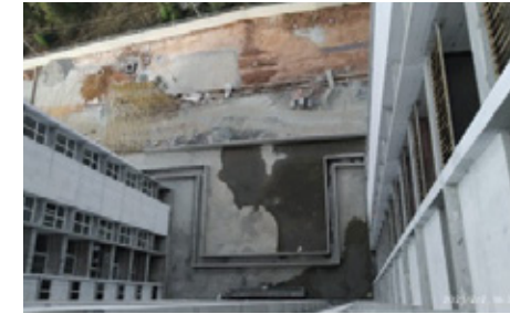
House Keeping (63° East - Tower D)
