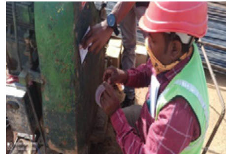
RCCB & Earth Pit Checking
