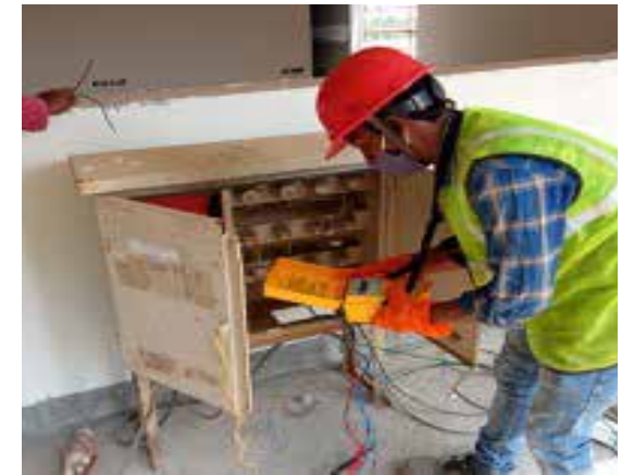
RCCB and Earth pit testing
