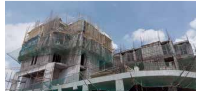
Vertical and horizontal periphery safety net fixing work in Tower B
