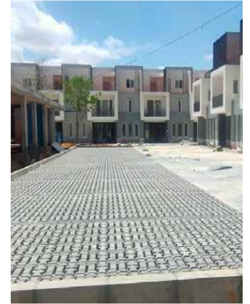
External car parking pavers work
