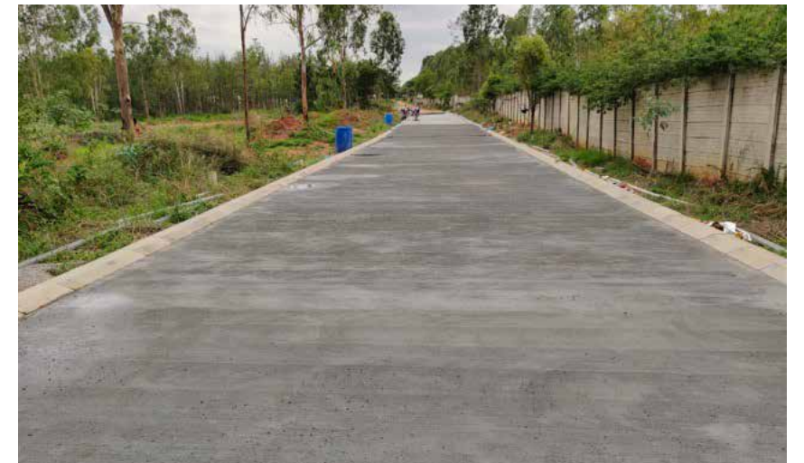
INFRA MAIN ROAD
