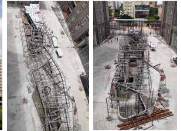
Entrance portal & central podium quadrangle roof ACP cladding work
