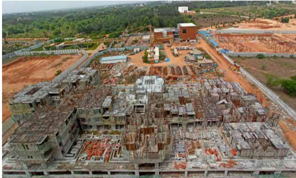
TOWER B – BLOCK B1, B2 & B3 AERIAL VIEW
